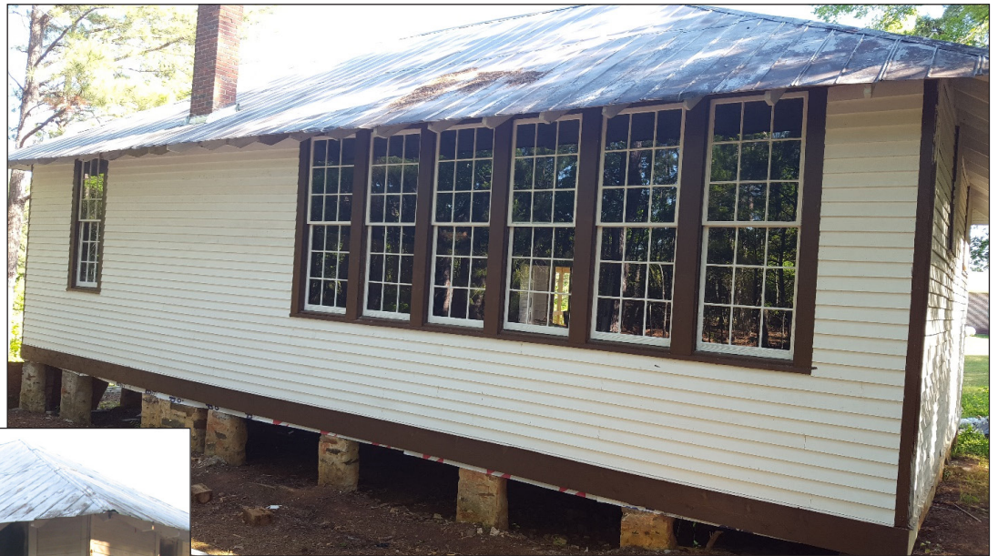
North exterior wall restoration. Photo to left shows the north wall and windows before restoration. Photo above shows the same wall after restoration, where the sill for the entire length of the wall was replaced.
