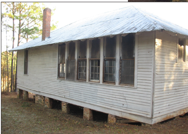
North exterior wall restoration. Photo to left shows the north wall and windows before restoration. Photo above shows the same wall after restoration, where the sill for the entire length of the wall was replaced.
