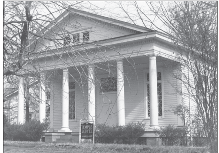
Temple Bethel, built in 1909 served the members of the Valley Jewish Community who primarily lived in the West Point-Bluffton residential area. The Temple was closed in 1963, purchased by a real-estate company in 1977, and later demolished.
