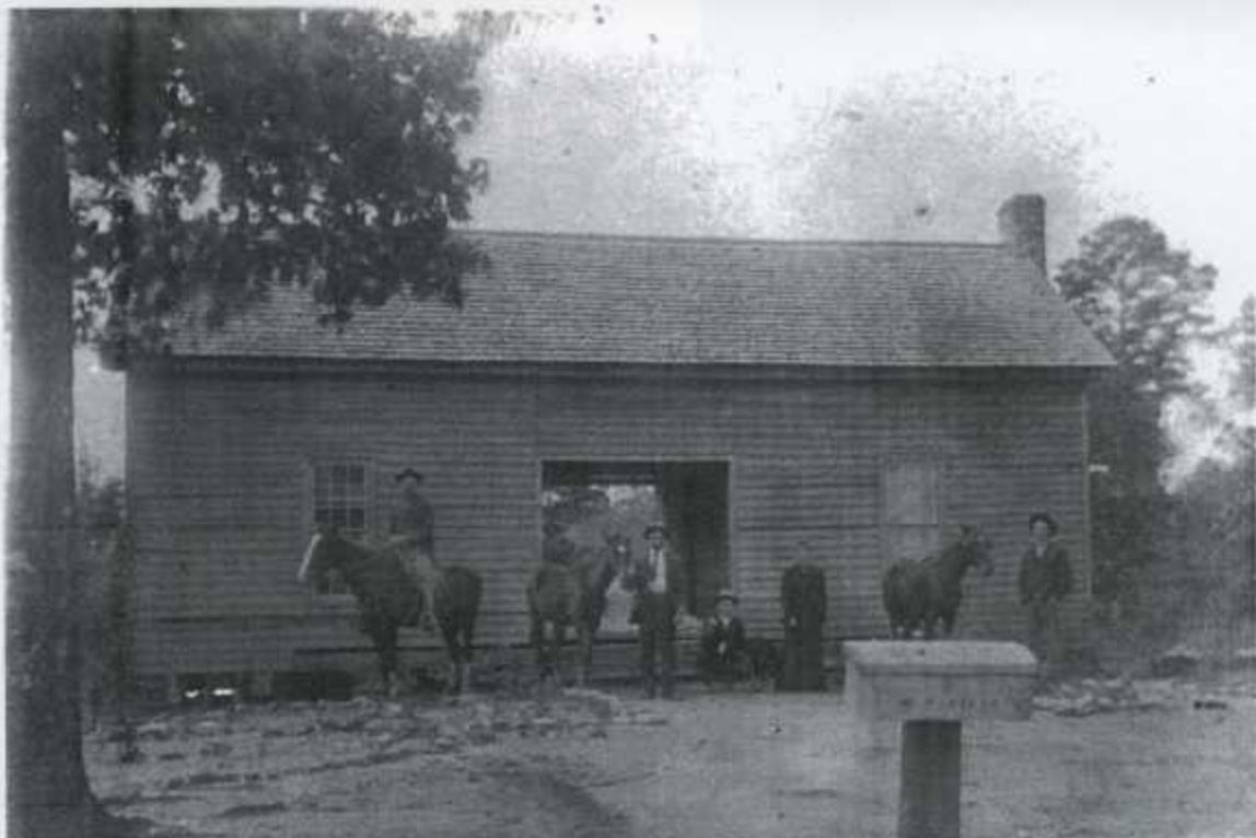
Located in the Hopewell community was the home of the W. W. Williams family. The open end hall referred to as a "dogtrot" was commonly found in rural dwellings. During the summer months it would be the coolest place to gather but unfortunately the same applied for cold winter days. After cotton picking time in the fall the family would pile cotton in the space until ready for ginning. Submitted by Ron Williams.
