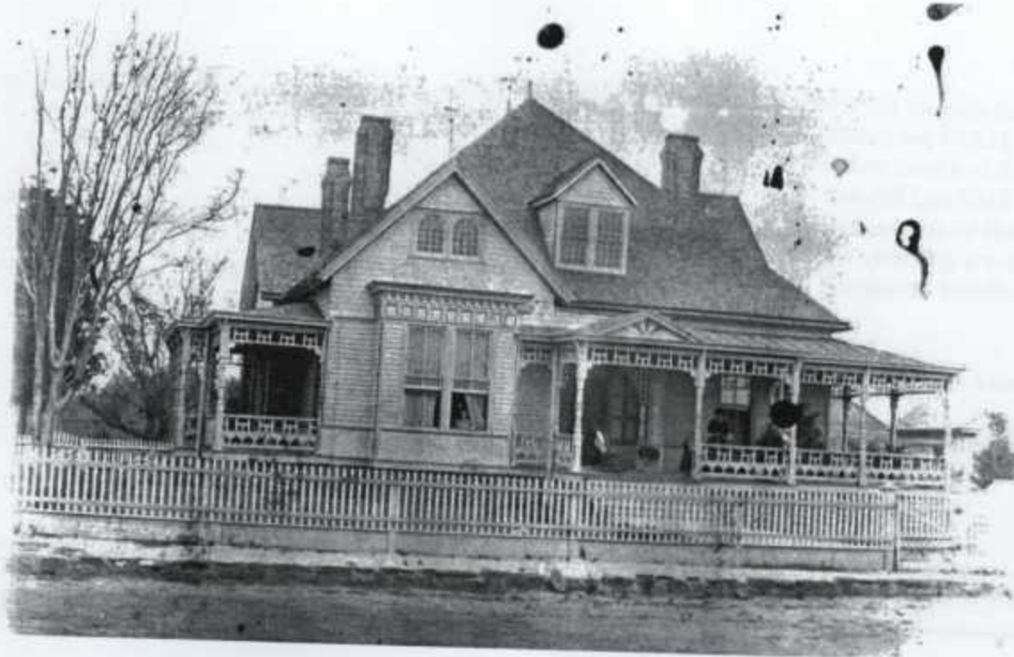
The Robinson House was built one mile east of LaFayette in the 1890s by Judge J.J. Robinson, Sr. and also occupied by the family of his son J.J. Robinson, Jr. when this photo was made. A fine example of high style Victorian architecture, the house and lands were later sold to the Hunter family. Hunter Subdivision, north of Hwy. 50, was developed from this property. Submitted by Betty Chambers Carr.
