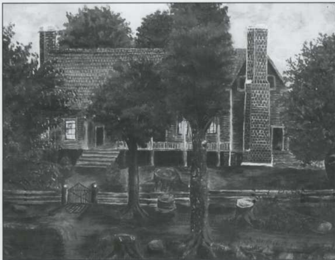
The Robert Floyd House was painted in 1877 by Margaret Josephine Combs (1857-1952) who was born in the house. Close examination of the painting reveals the 1 1/2 story Floyd House to have had two large rooms divided by an open hall or dogtrot. A shed room appears to be at the left end of the porch. Sleeping rooms above the two large rooms downstairs received light and ventilation from window openings at each side of the chimneys in the gable ends. Houses of this design were very typical of the plantation architecture used in antebellum Chambers County.
